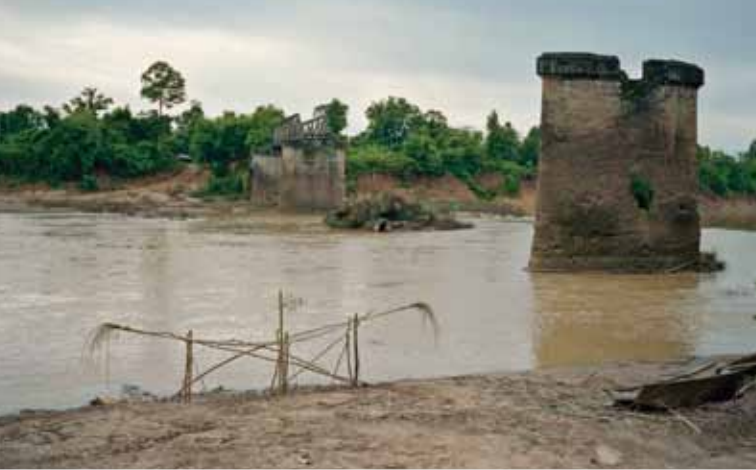
Khoua Ban Darn Broken Bridge, remains after bombing during Second Indochinese War
